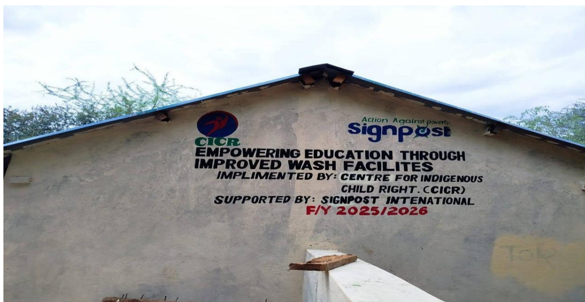
Toilets (4 per school * 2 schools = total 8) constructed under WASH (funded by Signpost International) at Primary Schools in Nakwijit, West Pokot. 2025
